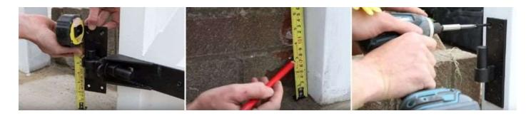
Once you have both hinge plates connected to the post, take a straight edge (long length of timber – may need two together) and span across the opening. Place a level across and mark the position of the hinge plates on the opposite post. Mark holes and screw hinge plates.
