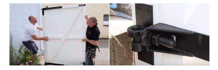
Once both sides are hung, adjust the hinges using the two bolts to align the height and sides. Each side should have an equal gap width with the centre being 10mm. Can take a bit of time to get exact. The gate should now be able to swing open and close freely.
